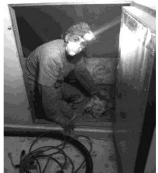
Installation work by Energia worker.
